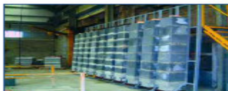
Photo 4 New system - factory assembly
