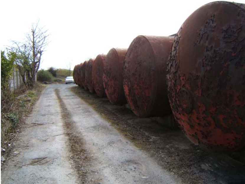
Figure 1-3. Pressure Filters at the now closed Terryland Old water treatment plant in Galway City.
