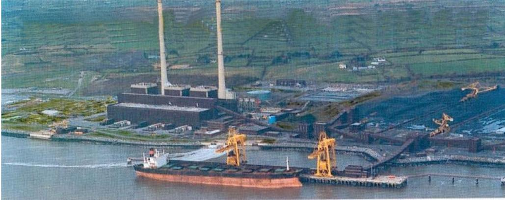
The plant has three generating units of 305 MW<sub>el</sub> each, even though the original design envisaged the construction of a fourth 305 MW<sub>el</sub> unit and both 220 metre high chimneys are each capable of serving two such units. All units are dual fired capable of full load on coal and/or HFO firing. Coal is the primary fuel with approximately 2 million tonnes consumed per annum. The resulting ash from the coal burning is presently land filled on-site.
