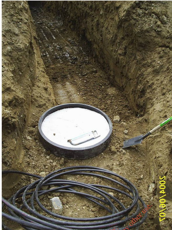
The lysimeter is secured by placing the clay firmly around the system.
