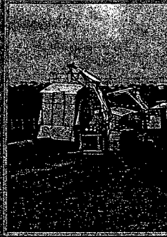
"Train" of automatic weld each completes one weld
