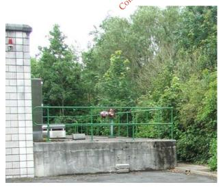
The Inlet Pump Sump consists of a two level tank internally with the incoming flows discharging to the deeper section of the Tank (2.3 mOD Malin Head).
