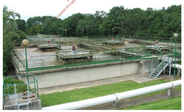
Each stream has a Primary and Secondary Surface Aerator (1 No. 45 kW, on inverter, and 1 No. 22 kW respectively) with a combined design aeration capacity of 75 kg  $O_2$  /hour. (This figure is accepted although no calibration data from installation was available.)
