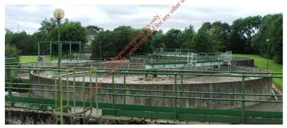
Due to the lack of a selector tank or anoxic zone in the biological treatment section of the Plant there would be a susceptibility to denitrification occurring in the clarifiers giving rise to excessive scum.
