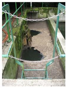
Final Effluent Inspection Chamber. A new manhole / chamber should be constructed to facilitate the operation and maintenance of such a meter.
