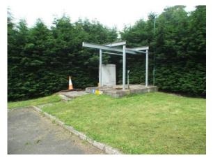
There are regular maintenance problems with this pumphouse due to blockages of the pumps by ragging. This is an increasingly common phenomenon around the country in recent times and may be due to the advent of the more fibrous kitchen and toilet papers. A maceration system, such as the Mono Muncher type, is recommended ahead of remote pumping stations to address this problem.
