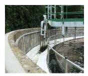
If the Hydraulic Load is increased to 17,280  $m^3/d$  the loading rate would increase to 27.5  $m^3/m^2/d$ . This is still an acceptable loading rate and should not compromise the effluent standard, although it will become much more important to control the type of bacteria in the process system (i.e. prevent the growth of filamentous bacteria). Control of scum may also become a problem.
