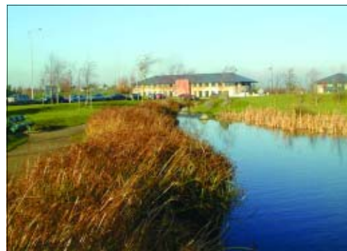
Balancing ponds, like this one, can prevent pollution, flooding, and also provide habitats for animals and birds.
