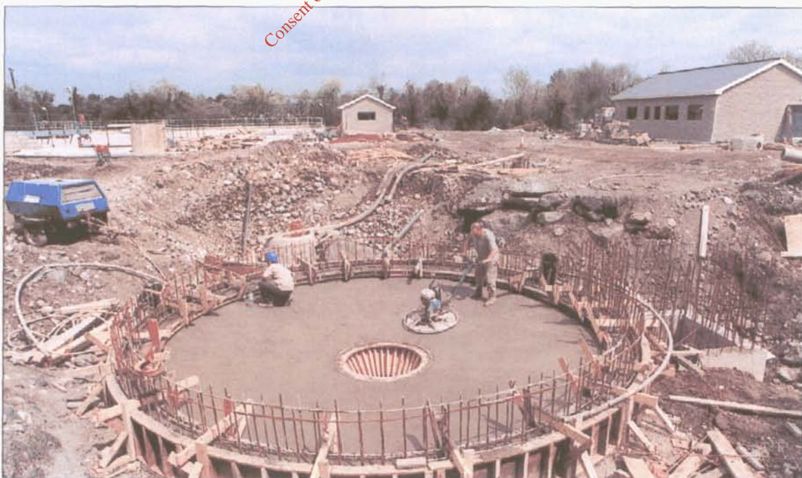
Construction of Secondary Wastewater Treatment Plant, Moate
