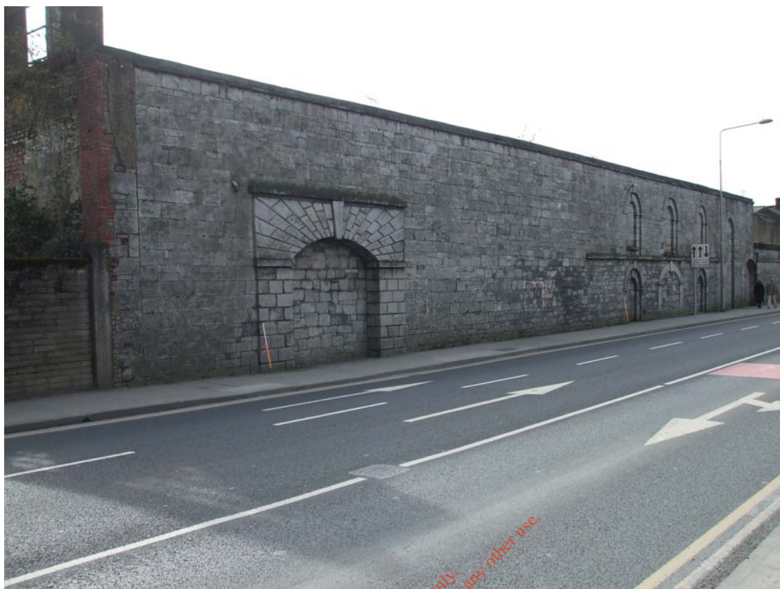
Plate 9. Exterior of boundary wall at Dock Road.
