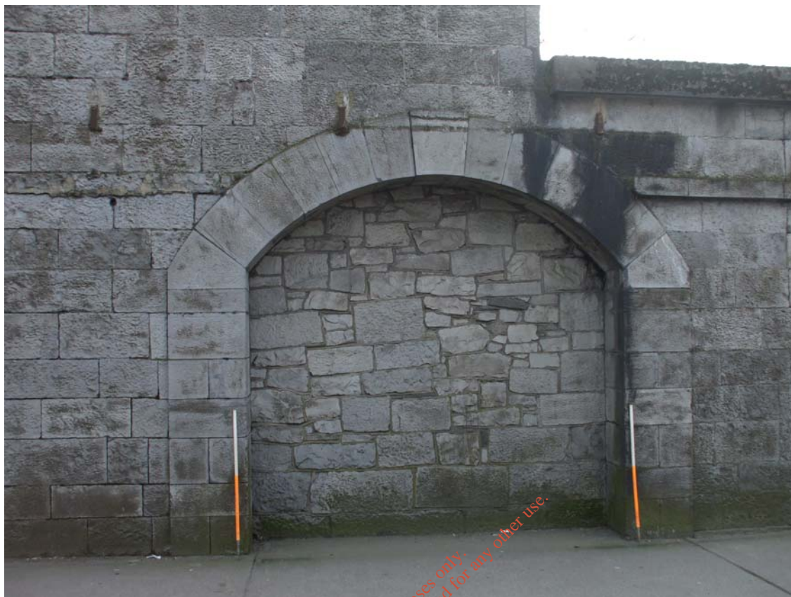
Plate 11. Blocked up segmented archway on Dock Road.
