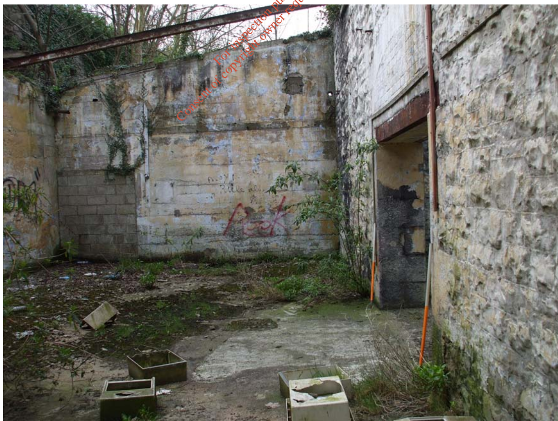
Plate 14. Rear section of Gasworks building.
