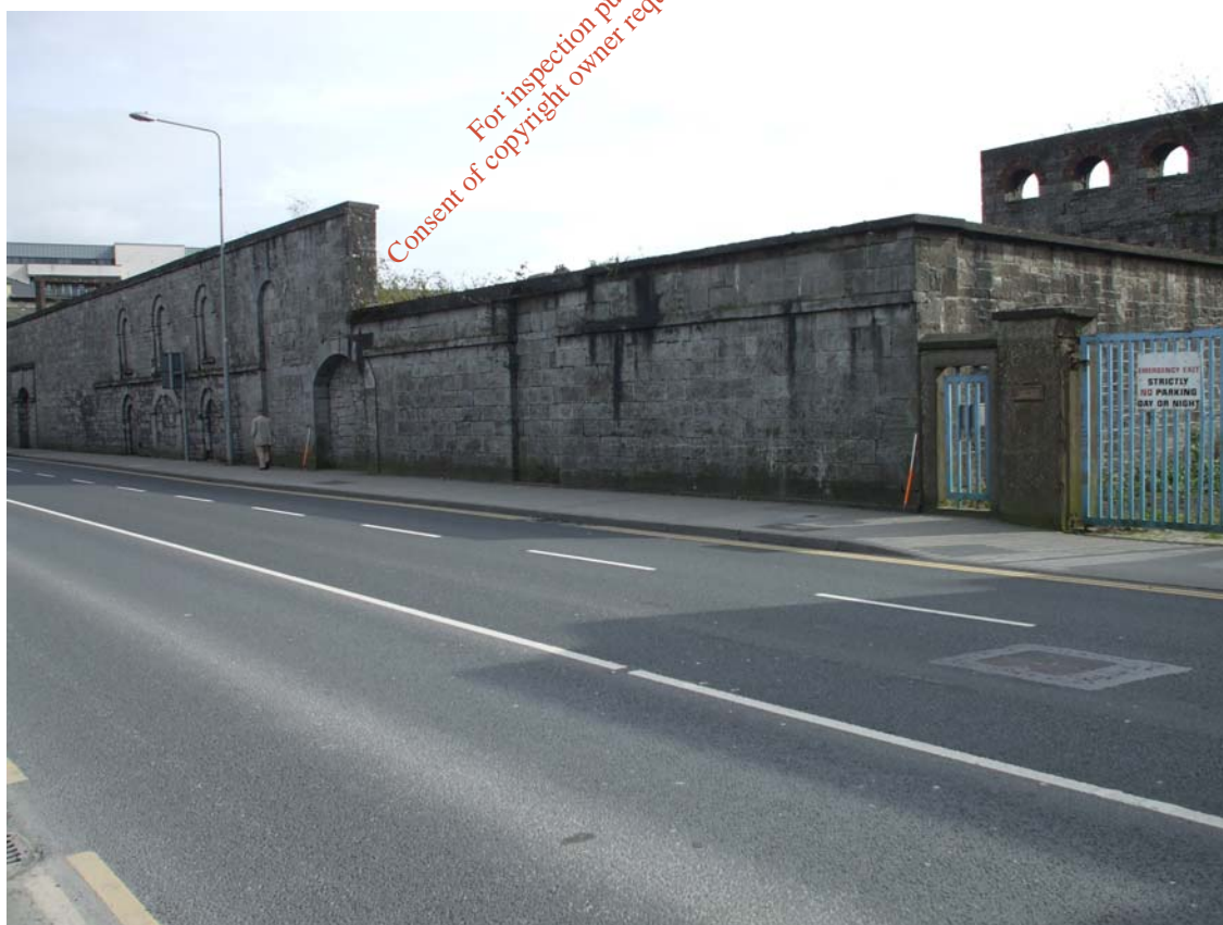
Plate 10. Exterior of boundary wall at Dock Road.
