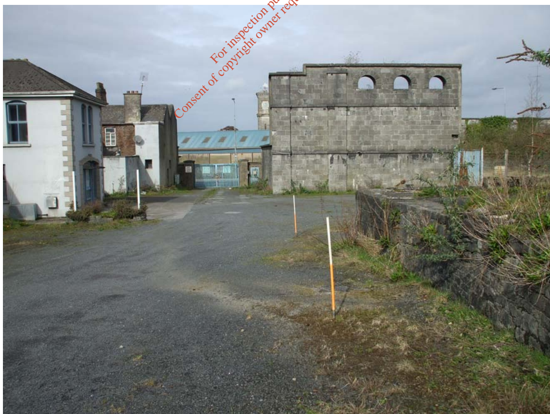
Plate 6. Interior of Gasworks facing north showing interior of boundary wall.
