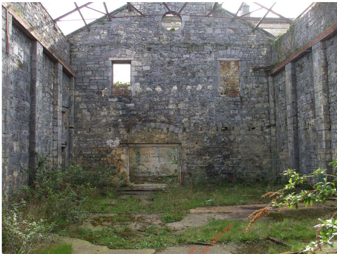
Plate 13. Interior of Gasworks building.
