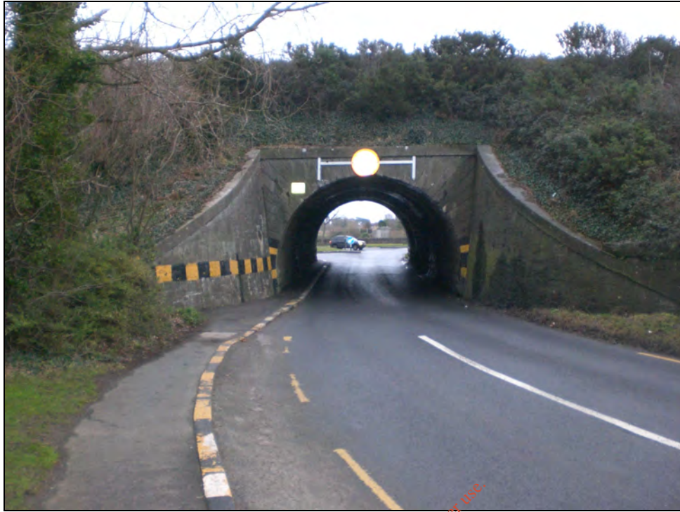
Plate 12.1 Low Rail Bridge along R127 on Approach to Skerries
