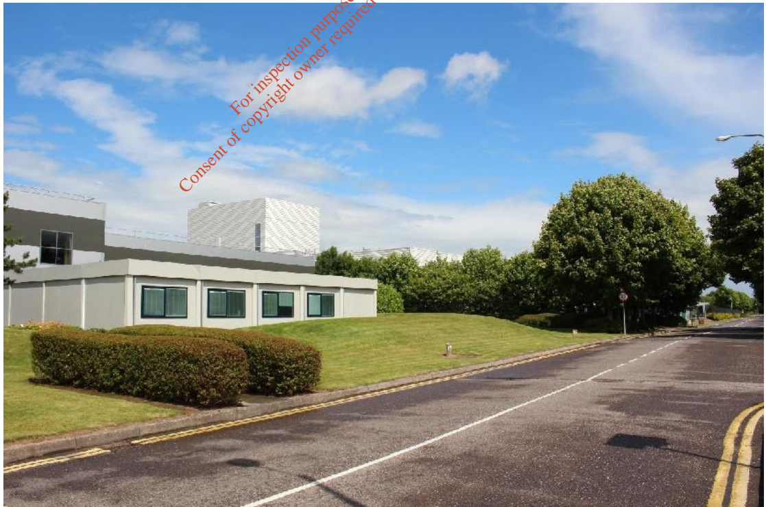
Plate .1 Photomontage view o proposed development See Appendi .2 or montages at A3 scale
