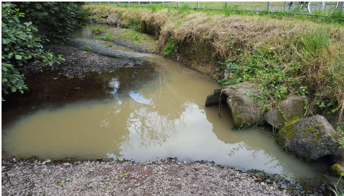
Photo 3. Discharge pipe from the Curraheen Pumping Station. Low flows at the time the photo was taken.
