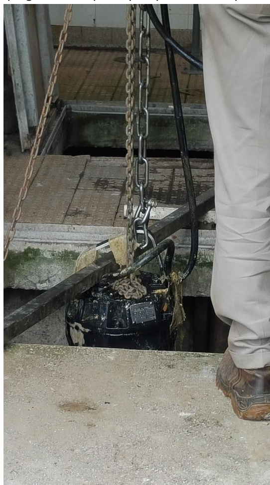
Photo 4. Curraheen Pumping station repairs, pump raised to replace seal.
