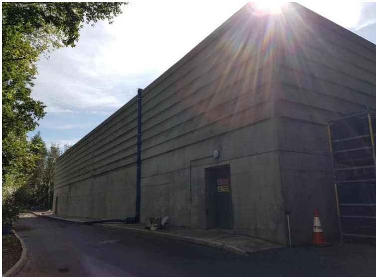
Photos 7 & 8 Redundant raw water balance tanks now in use to store supernatant allowing for additional settlement prior to discharge to Lough Corrib
