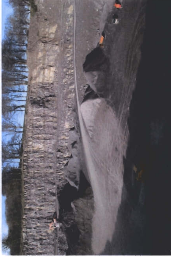
9. View of extraction area in Mc Tigue's Quarry – no evidence of any asphalt plant in site
