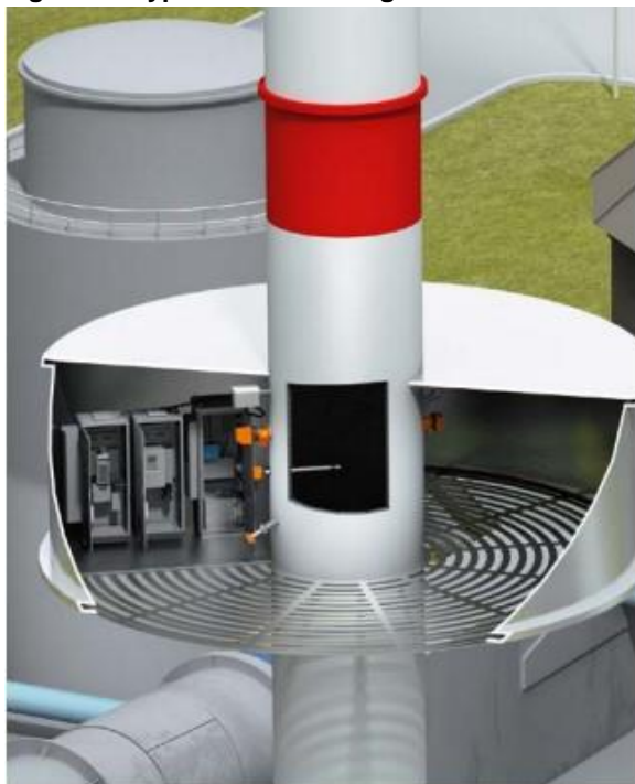
Figure 7 - Typical CEMS arrangement 11
