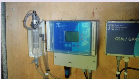
Chlorine monitor and alarm not operational
