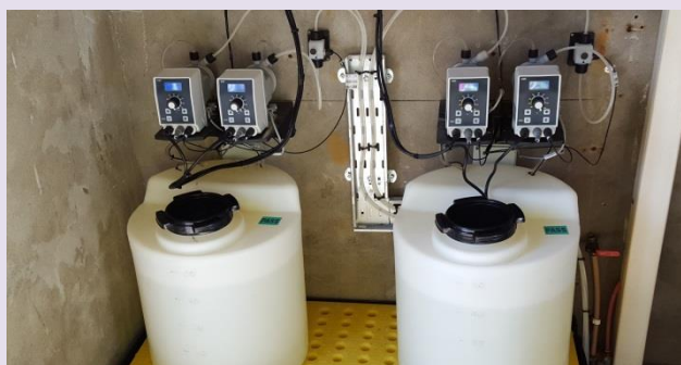
Duty/Standby dosing pumps with no automatic switchover
