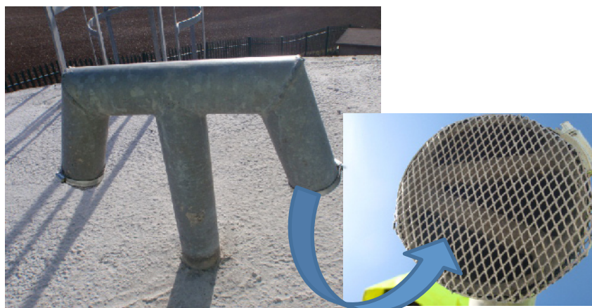
Adequately sealed reservoir vents preventing animal access
