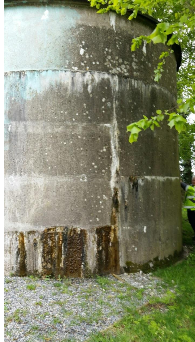
Photograph 3: Cracking visible on the side walls of Reservoir 1
