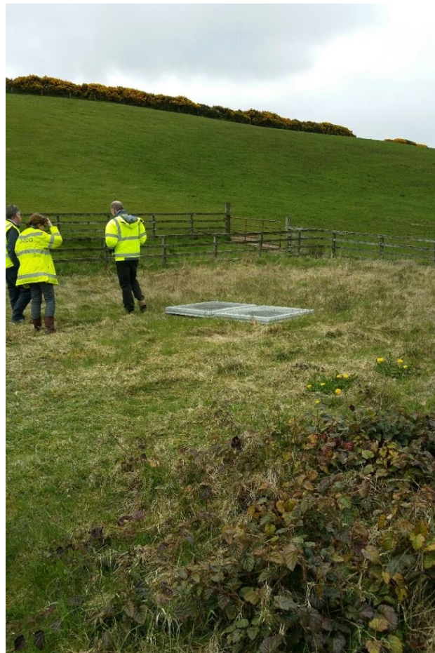
Photograph 2: Top of Reservoir
