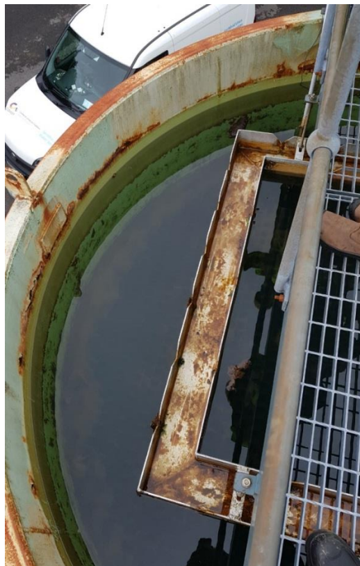
Photo 2 Sludge on channels and surface and rust on clarifier wall
