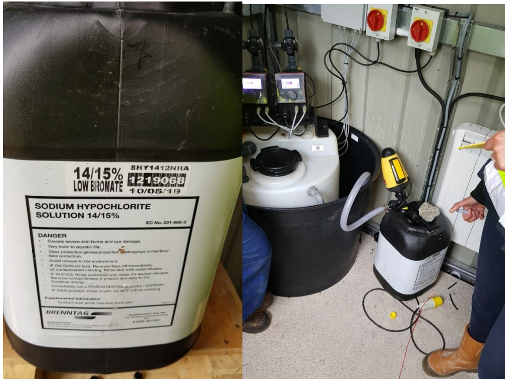
Photos 3 & 4 Drum of disinfectant labelled inappropriately and unbunded
