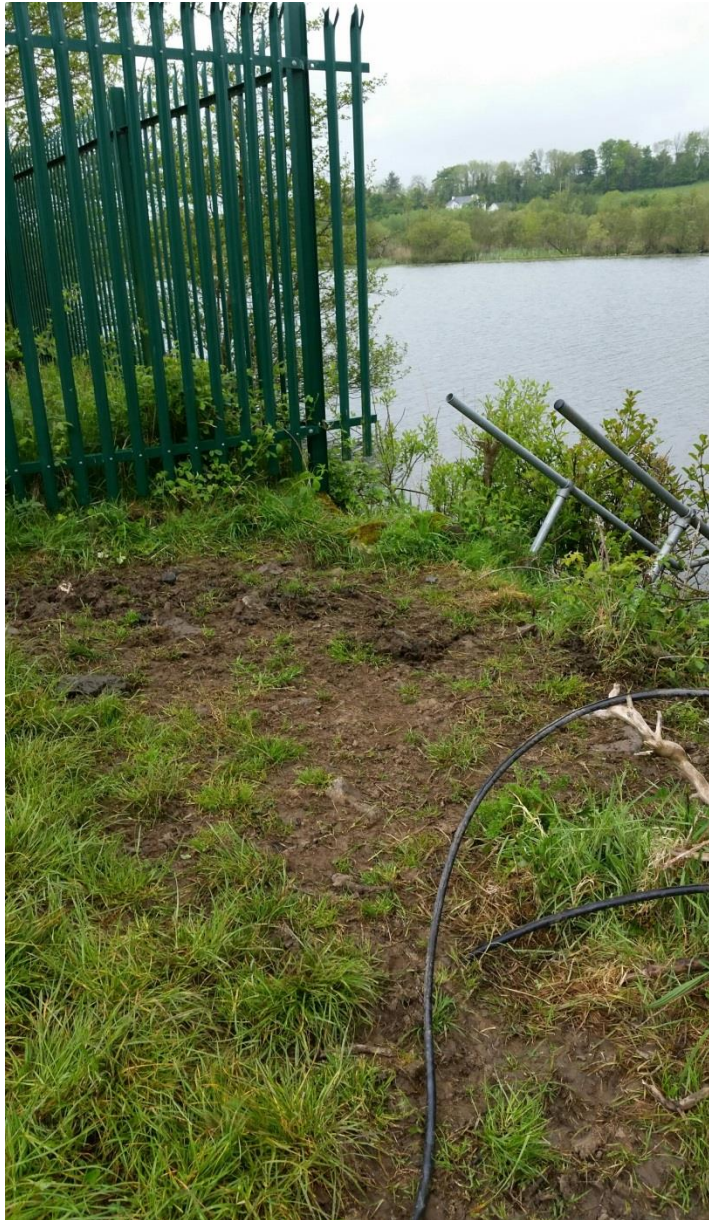
Photograph No. 1: Unfenced area of Coragh Lake shoreline adjacent to pumphouse palisade fence, showing cattle poaching and dung in foreground
