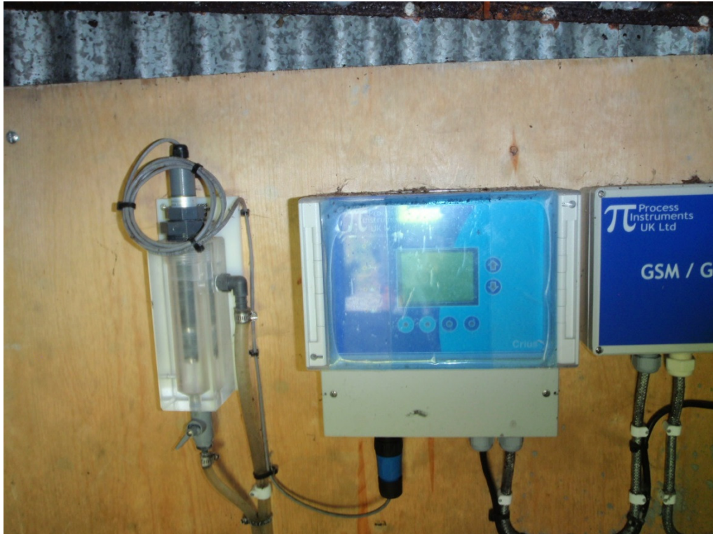
Photograph 4: Chlorine monitor at the Tulla reservoir (not operational).
