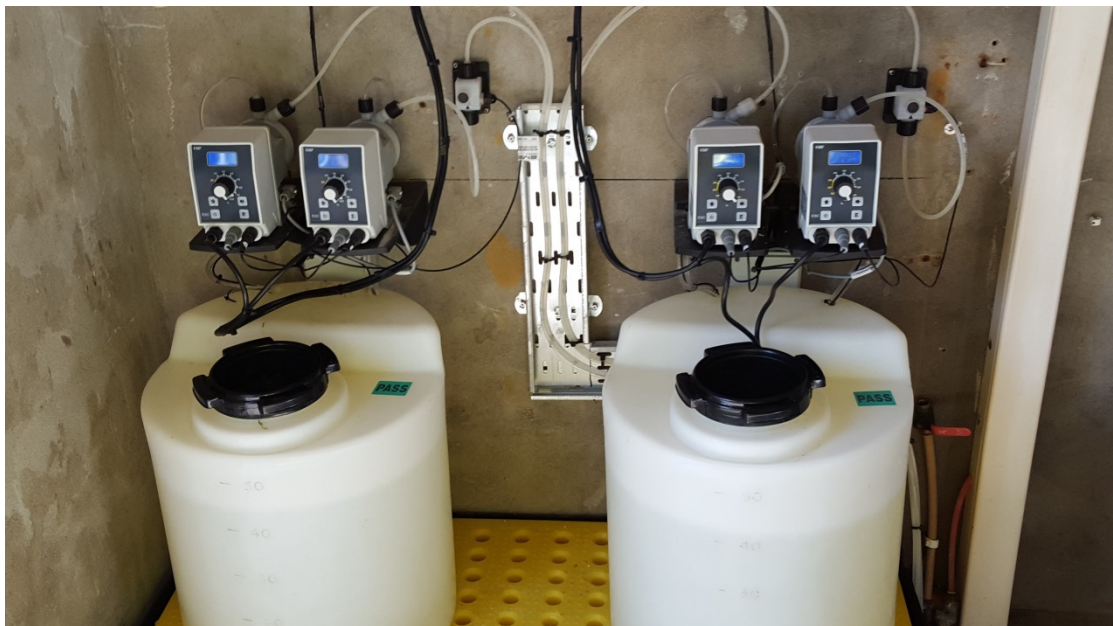
Photograph 2; Separate duty and standby pumps on the Broadford and Tulla supplies.
