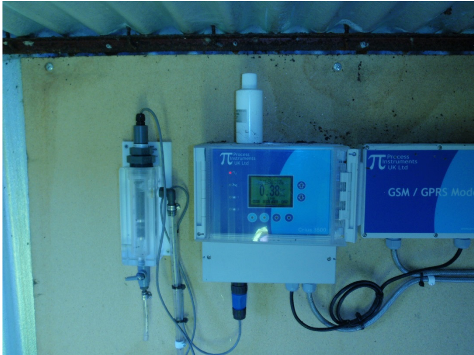
Photograph 4: Chlorine monitor at the Tulla reservoir (not operational).
