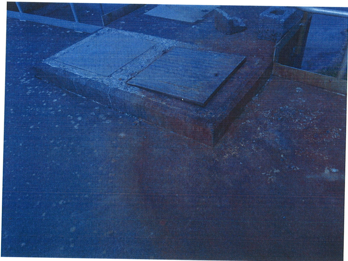
Photograph 4: Cover on ferric bulk tank not sealed and showing signs of spillage.
