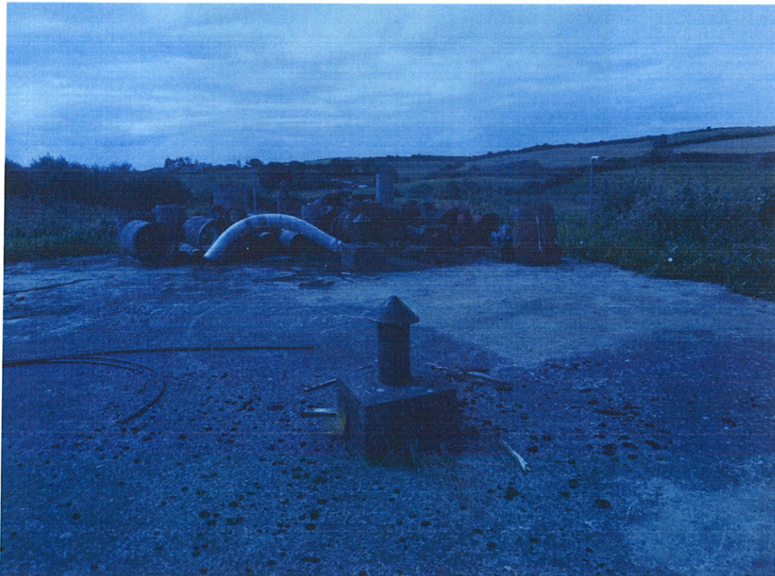
Photograph 8: Pipes and waste material stored on reservoir;
