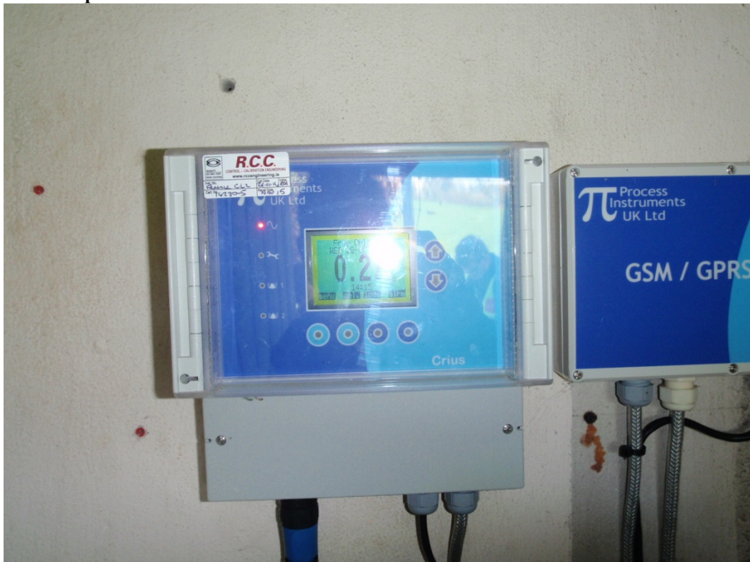
Photograph 2: Chlorine residual monitor located after the Feakle reservoir. There are no dial out alarms in place.
