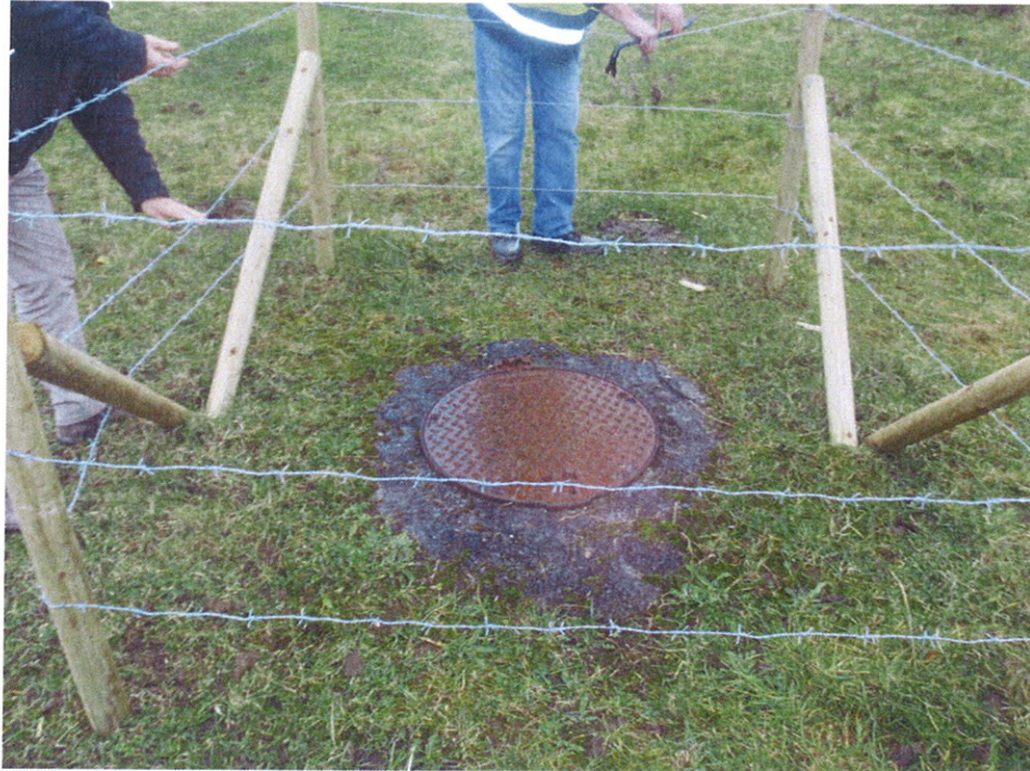
Photograph No. 1: Temporary fence around borehole. Head of borehole below ground level and chamber not of adequate construction.
