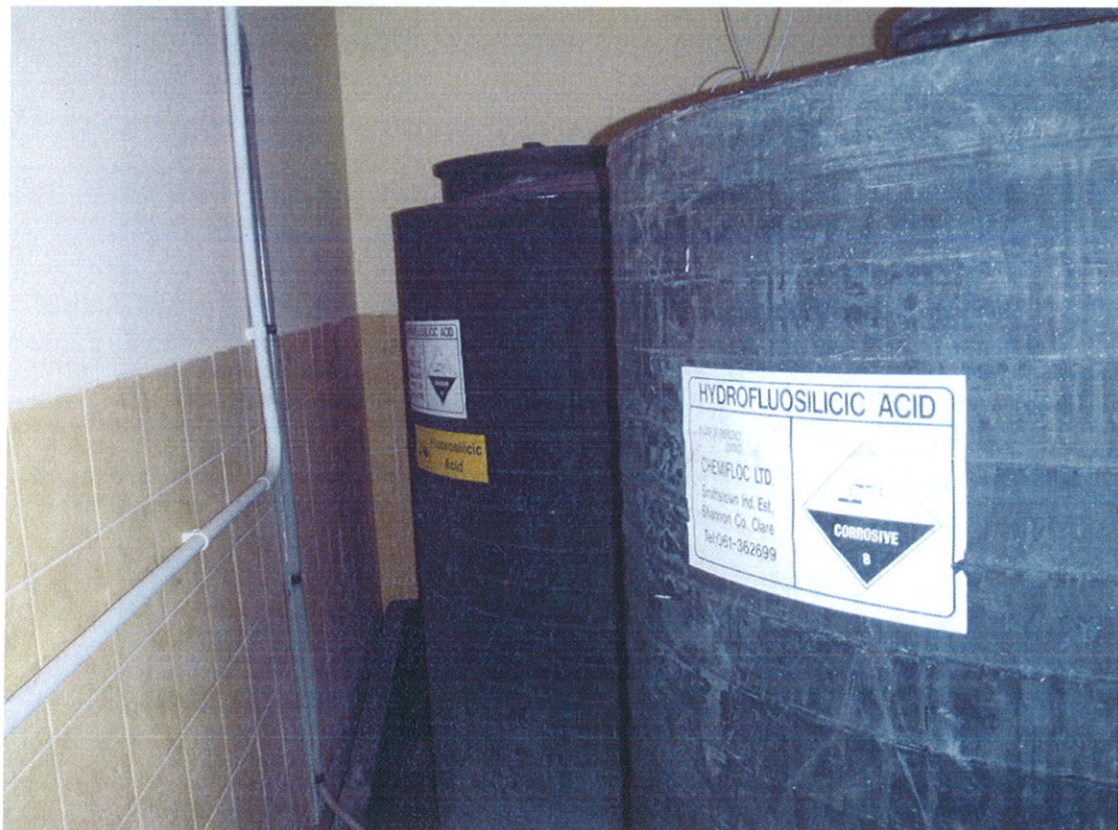
Photograph 6; Hydrofluosilicic acid bulk storage tanks.
