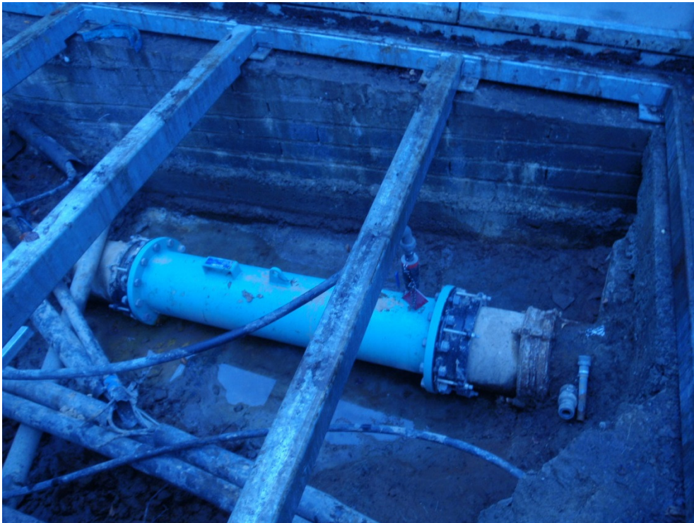
Photograph 5: No finished floor or sump within chamber, standing water observed.
