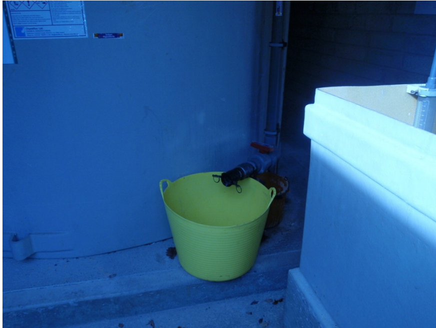
Photograph 4: Inappropriate spill tray on bulk storage tank.
