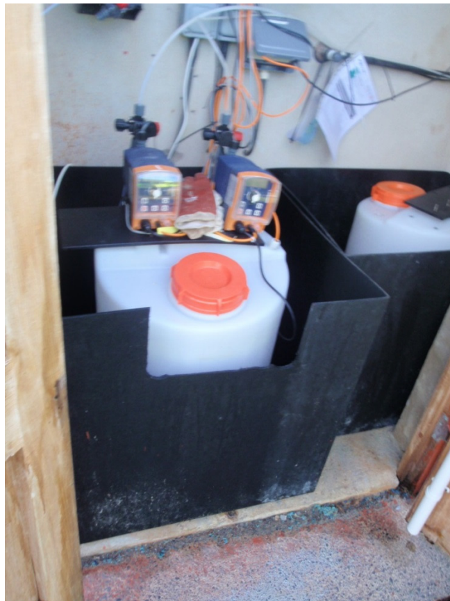
Photograph 3: Chlorine day tank adequately bundled.
