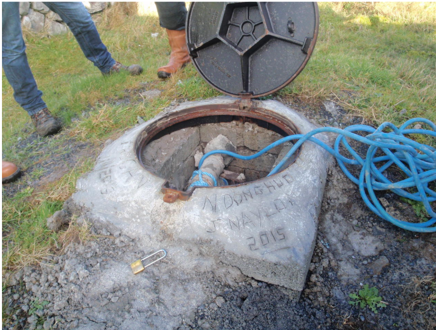
Photograph 2: Borehole construction not constructed as per EPA guidelines.
