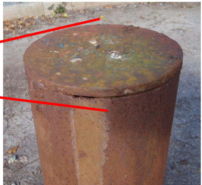
Photograph 2: Second borehole <10 m from operational borehole – unsealed and not decommissioned.
