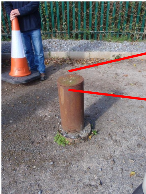
Photograph 2: Second borehole <10 m from operational borehole – unsealed and not decommissioned.
