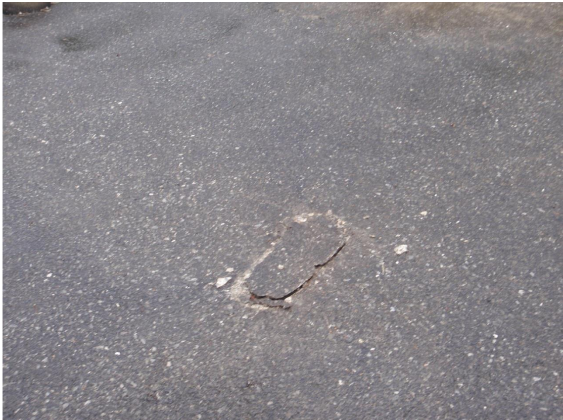
Photo No. 2 – Visible Damage on Roof of Clear Water Tank
