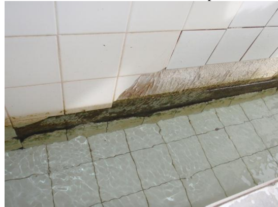
Photograph No. 2: Hygiene and Housekeeping: tilework on water channels in need of repair.
