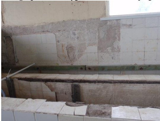
Photograph No. 2: Hygiene and Housekeeping: tilework on water channels in need of repair.
