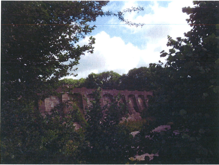
Photograph No. 1: The primary raw water source – an impounded lake located adjacent to the plant.
