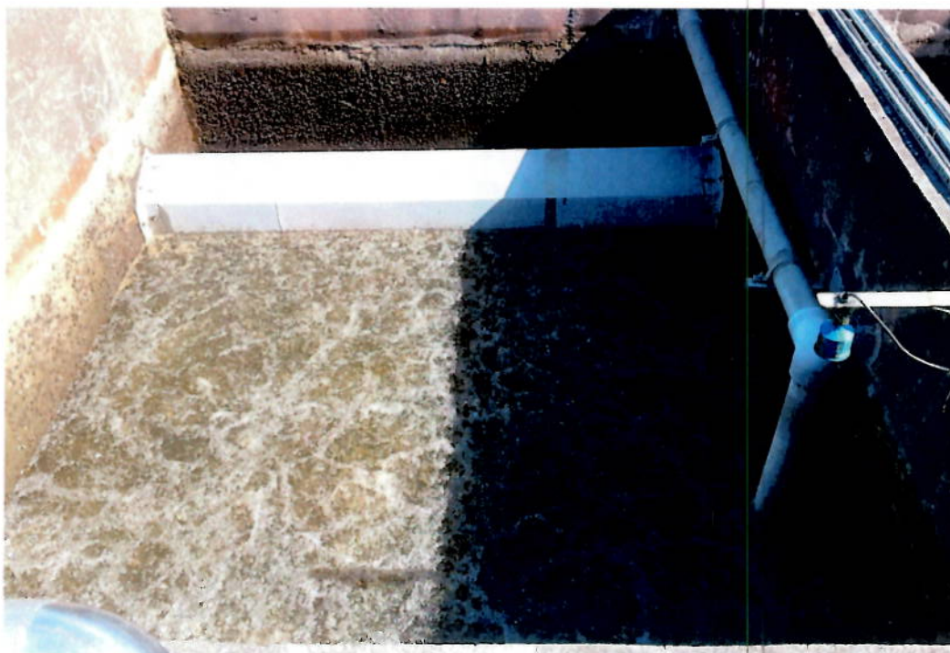
Photo 4 Even distribution of backwash water on Filter No. 3
