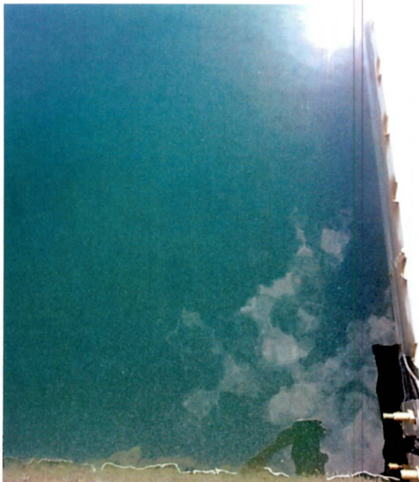
Photo 3 Pin-floc evident in clarifer
