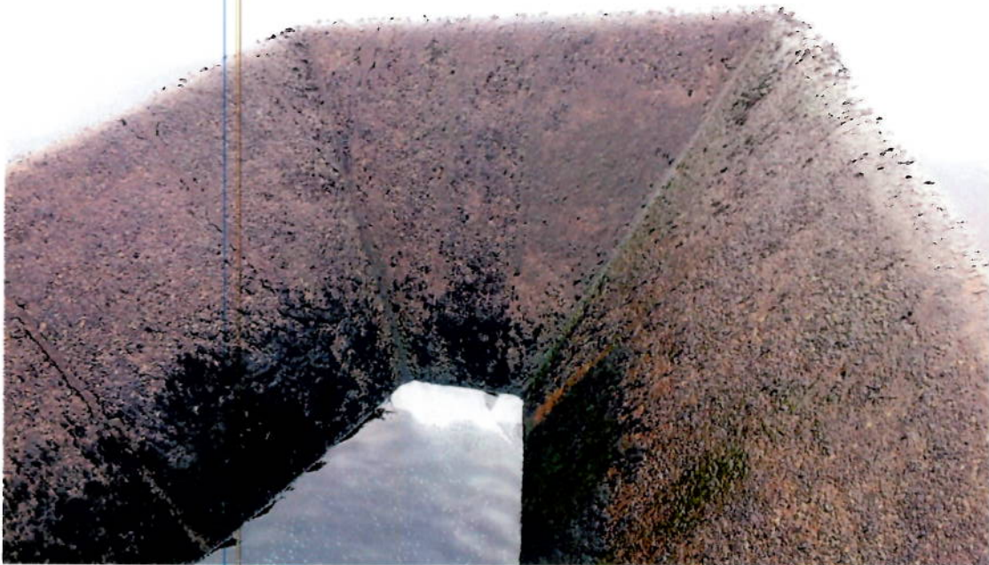
Photo 3b Overflow weir at Lough Keel
