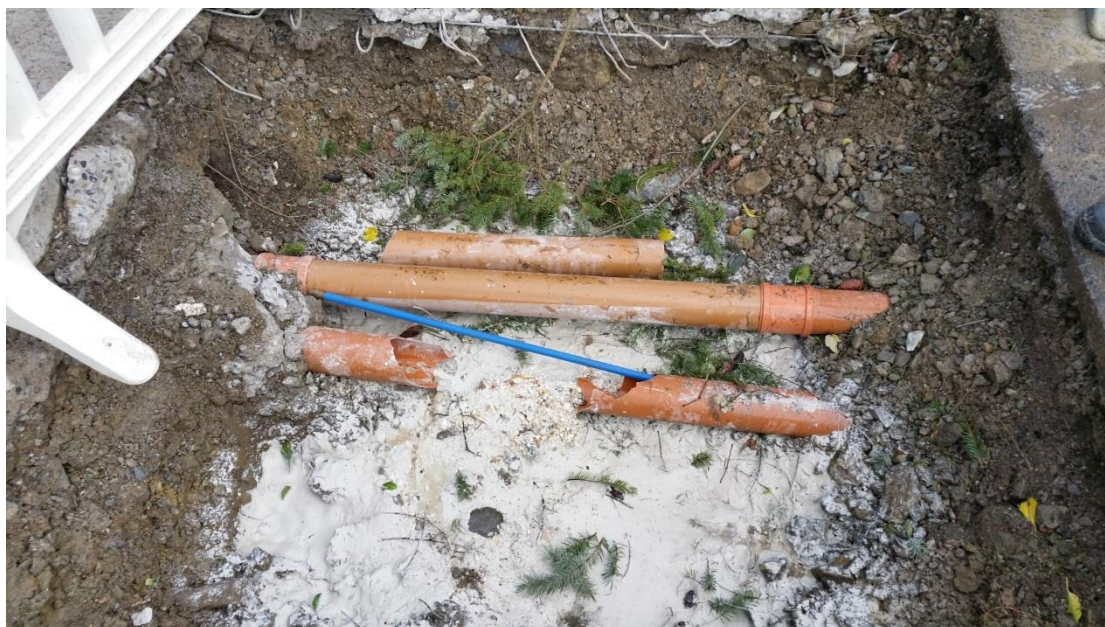
Photograph 1: Remedial works to lime slurry drainage and surface water drainage pipes.
