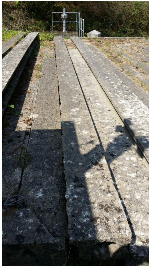
Photo 1. Cover of the Callow Hill Break Pressure Tank
