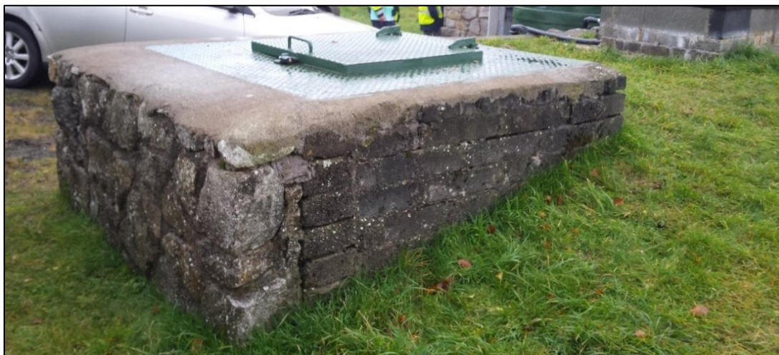
Photo 1: Borehole chamber at Glencullen water treatment plant
