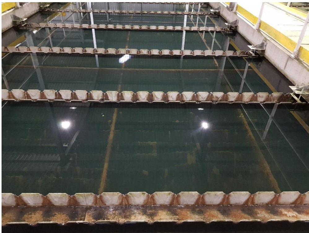
Photo 1: Clarifier in poor condition with visibly damaged/collapsed lamella plates at MMcP plant
