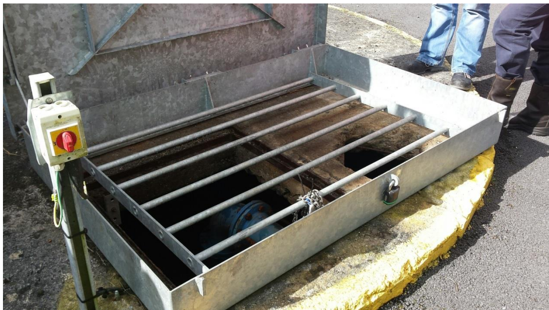
Photo 2: Spring abstraction chamber
