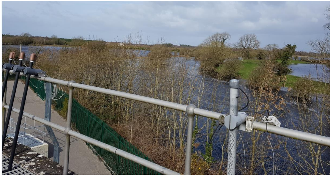
Photo 1 River Suck and Bunowen River burst its banks - water surrounds perimeter of water treatment plant due to flooding
