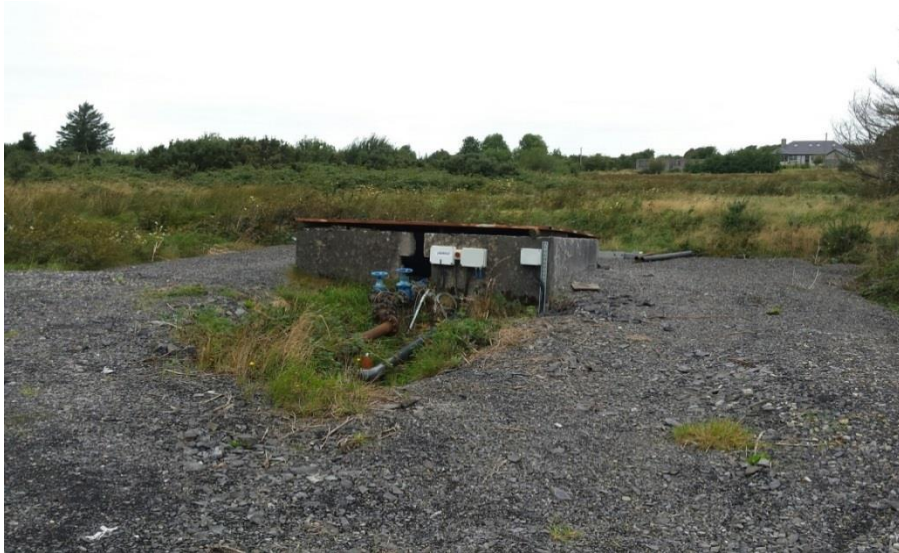
Photo 1: Bushtown spring chamber - refurbishment works to be completed
