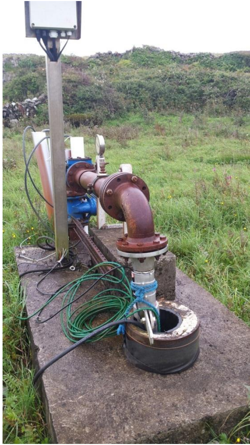
Photo 3: Uncapped borehole
