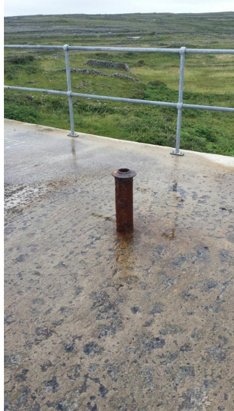
Photo 4: Open vents at Kilcarna treated water reservoir
