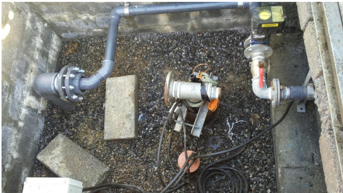
Photo 2: Plant borehole needs to be decommissioned
