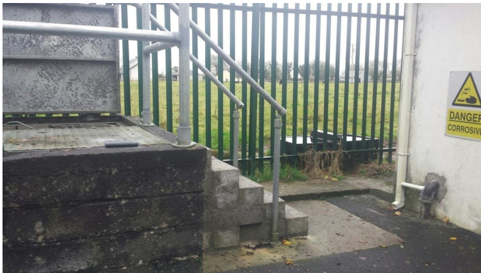
Photo 2: Proximity of water trough in adjacent field to the borehole chamber.
