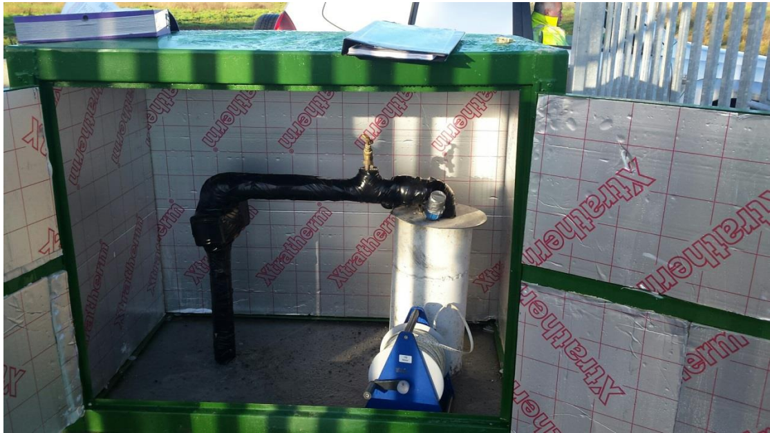
Photo 1: High standard of wellhead protection at the borehole source
