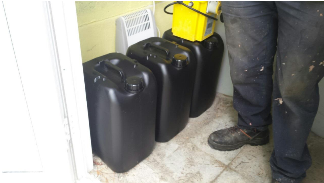
Photo 1: Sodium hypochlorite drums stored in an un-bunded area
