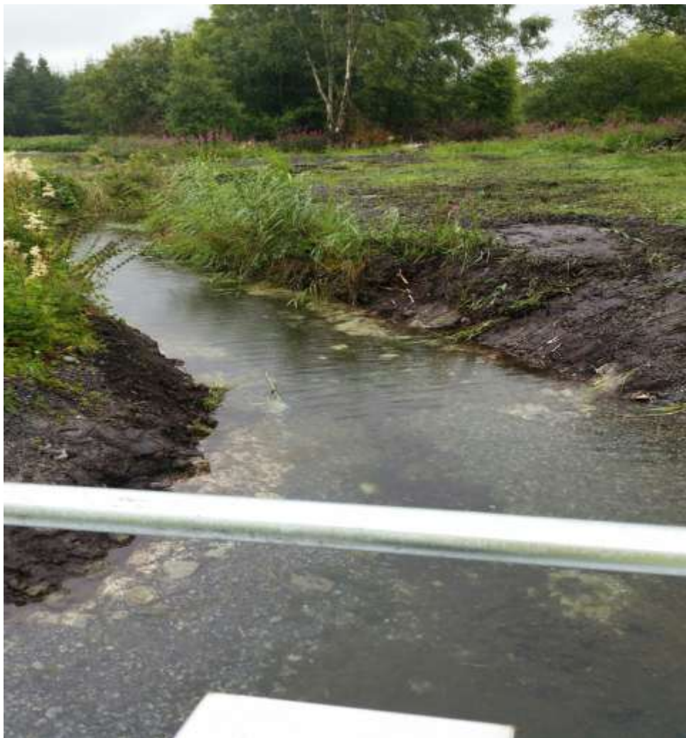
Photograph No. 1 Cleared vegetation around spring source and river
