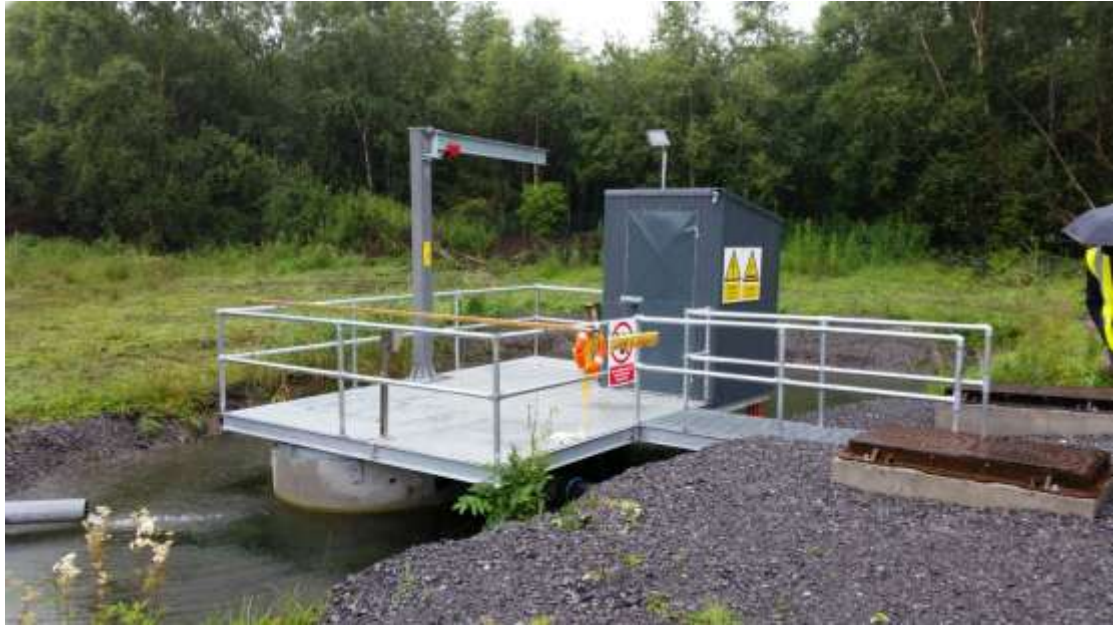
Photograph No. 2 Cleared vegetation around spring source
