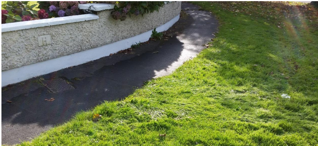
Photo 2 Grassy area in Moyola park where hydrant drains flushed water to.
