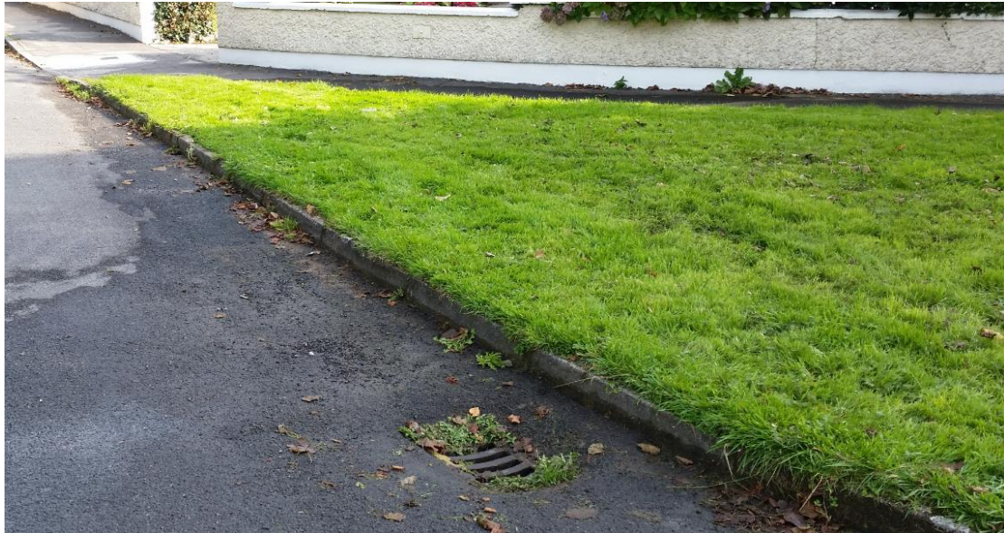
Photo 1 Grassy area in Myola Park where hydrant drains flushed water to. It was unclear if flushed water eventually drains to a surface water or waste water outlet.
