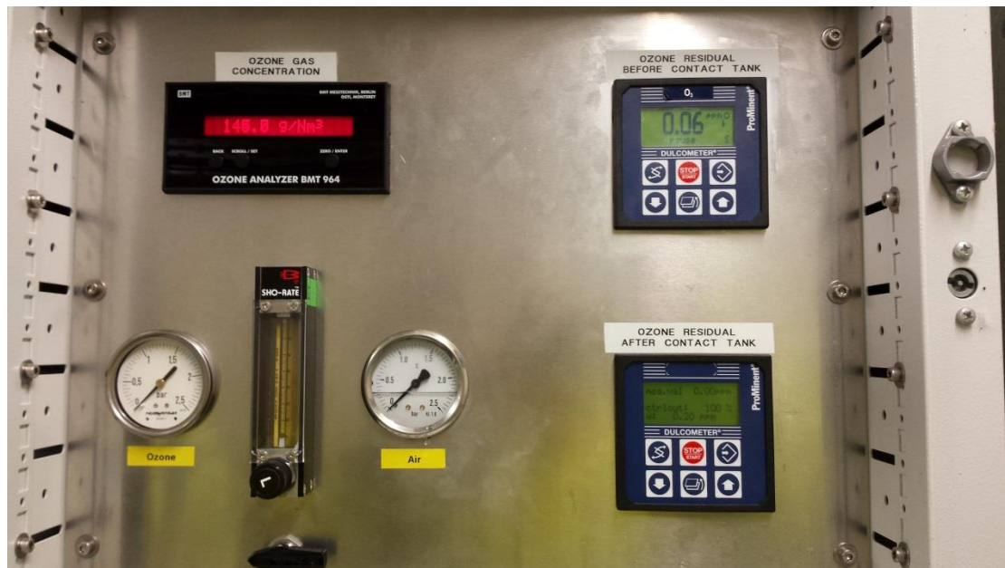
Photo 1. Ozonation Panel (note Ozone Residual After Contact Tank is 0.00 ppm)
