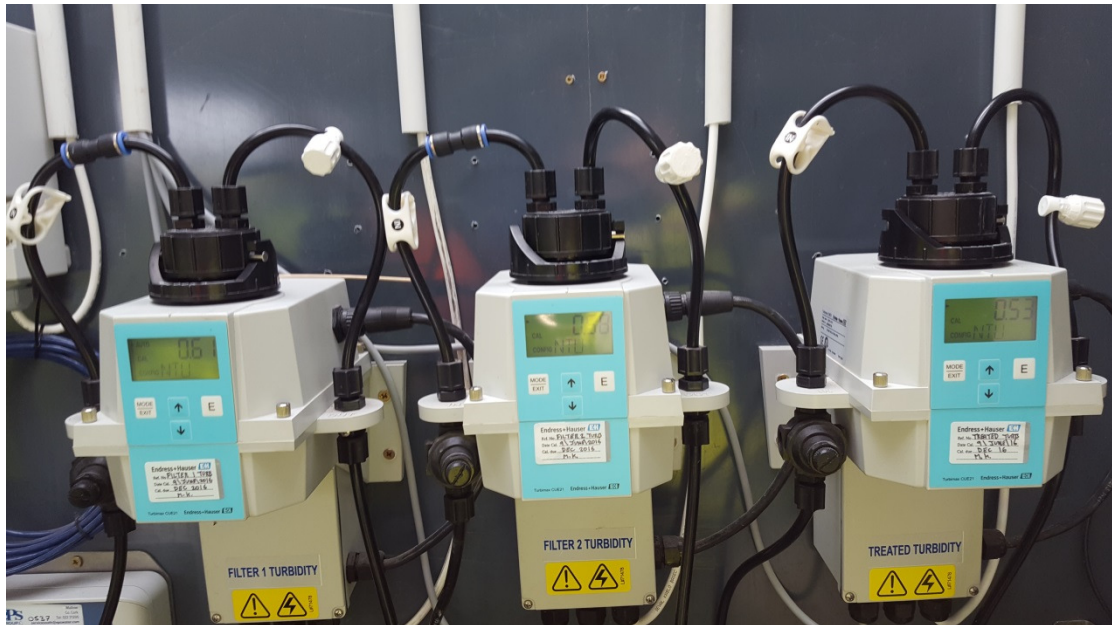
Photograph 1: Turbidity monitors, with results > 0.2 NTU. Readings from filters 0.61 NTU, 0.58 NTU and reading in contact tank, 0.53 NTU.
