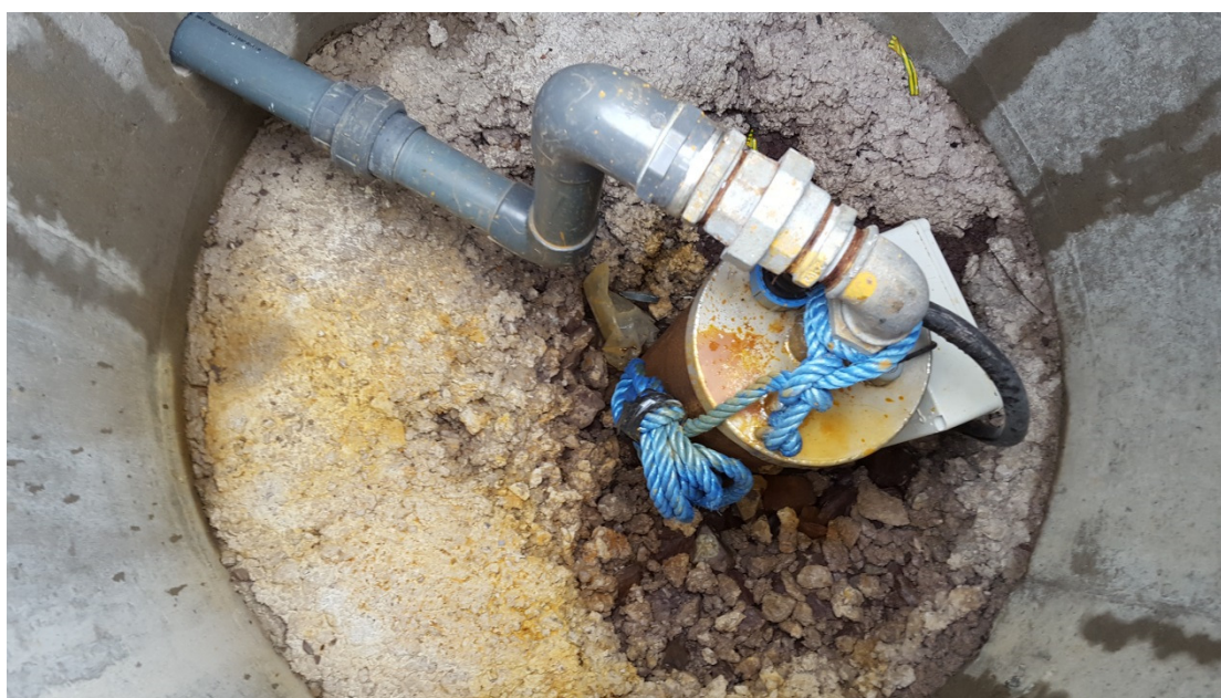
Photograph 1: Borehole head adequately sealed and protected.
