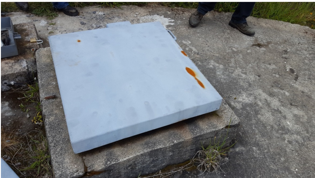
Photograph 4: Appropriate covers on reservoir to stop contamination and insect ingress.
