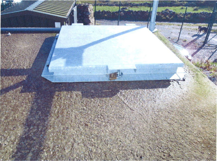
Photograph 3: Sealed and lockable covers were on all hatches.
